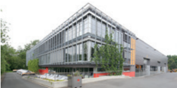
The development and sales centre with assembly halls of Müthing GmbH & Co KG Soest.
